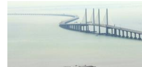
Penang Second Bridge (around RM4.5bn)
